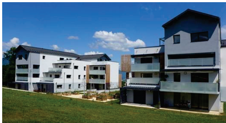
Figure 3. Residence Les Roches Blanches, source: Jean Paul Faure Architect.
